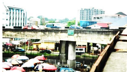
Mile One Bridge
